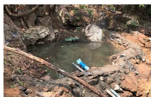
Community members working together to install water pipelines
